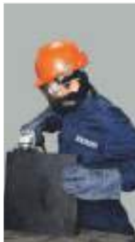
Finishing Bearing Pad
