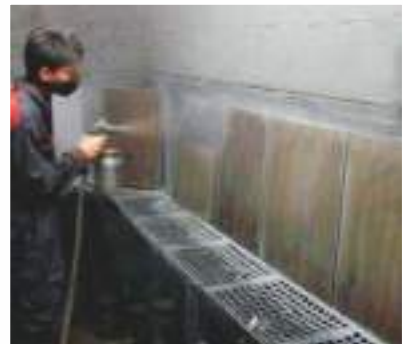
Plate Preparation with Bonding Agent
