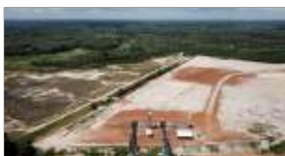
Proyek Underpass Desa Tenam Jambi
