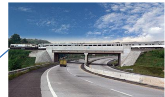
Bridge & Toll Road Cipularang
